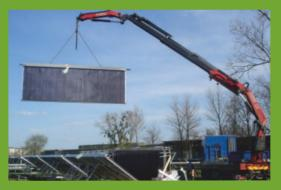
Structure of the MEGA collector segments with 78 tubes for a large solar collector field
