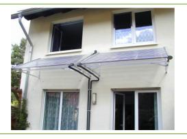
**place:** single-family house, Berlin, Germany **plant:** approx. 5 kW<sub>p</sub>; 50 direct flow Power tubes, 8m², 500 I storage, absorber 45° optimum, roof for
