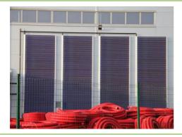
place: industrial facade, Kekava, Latvia **plant:** approx. 29 kW<sub>p</sub>, 45,2 m<sup>2</sup>, 280 direct flow Power tubes
