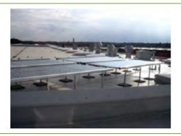
**place:** Logistic centre, Lehrte, Germany **plant:** approx. 25 kW<sub>p</sub>, 39,5 m<sup>2</sup>, 240 direct flow
