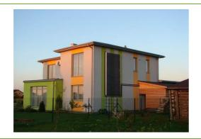
**place:** single-family house, Kekava, Latvia **plant:** approx. 6 kW<sub>p</sub>, 10 m<sup>2</sup>, 60 direct flow Power tubes, 10 m<sup>2</sup>, 800 I storage, absorber angle 60°
