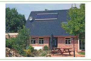
**place:** single-family house, Meppen, Germany **plant:** approx.  $6 \text{ kW}_P$ ,  $9.8 \text{ m}^2$ , 60 heat pipe tubes **application:** domestic water heating and heating support
